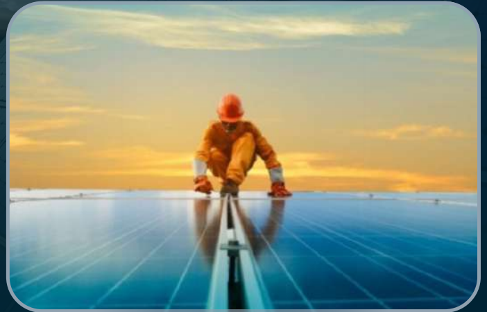
Photovoltaic installation maintenance
